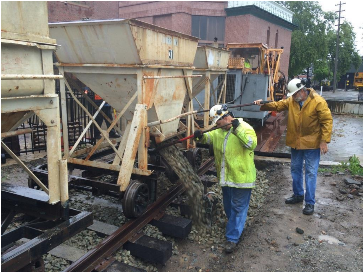
Mike F. and Alan ballast the track using the side-dump ballast hopper. Chris skillfully controls the motion in the tamper
