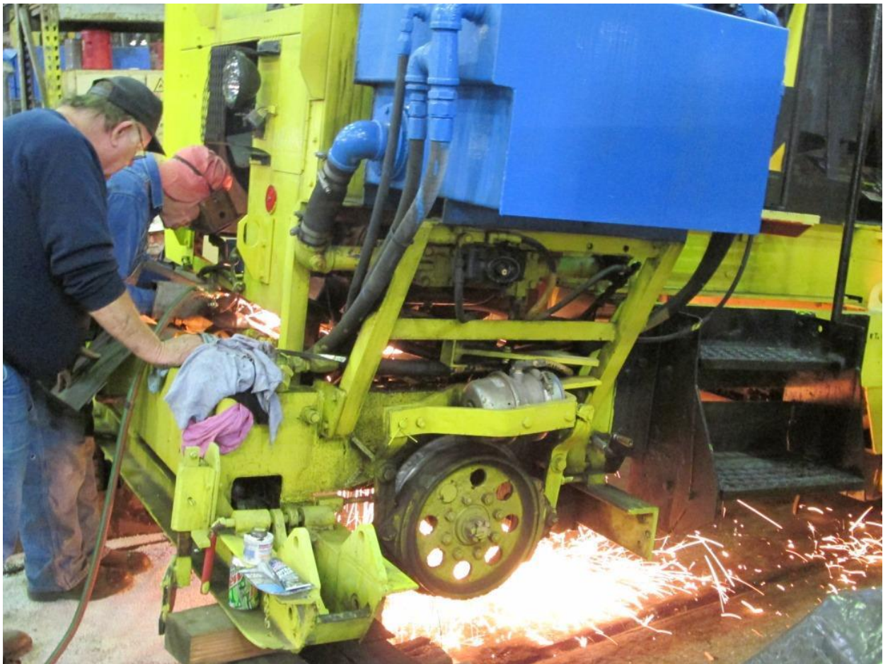
Cliff cuts away a part of the frame of the man-lift with Gene's assistance
