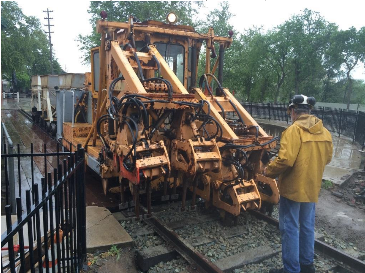
Let the tamping begin. Chris in the tamper tamps the first ties under Alan's direction
