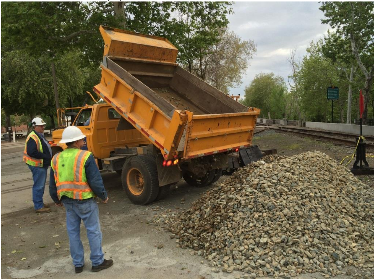
Frank driving the dump-truck while Chris and Mike H. give direction
