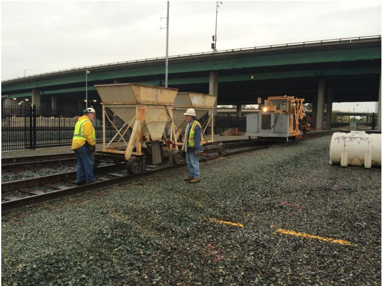
Conductor Frank and Mike M. gather the ballast hoppers using the tamper to run them over to Old Sac.
