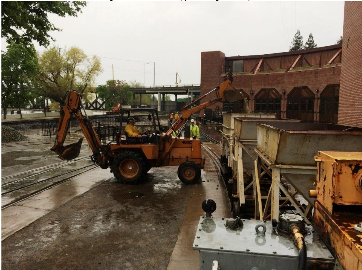
Now spotted on the dual-gauge track, Harry in the back-hoe loads the hoppers with rock
